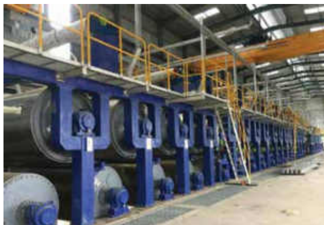
A view of paper machine under installation
